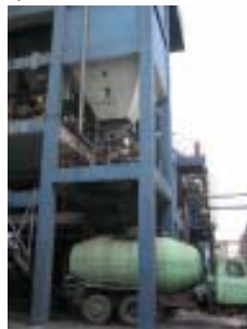
Steam cooled cyclone (above 100 T/H capacity) Power Plant use Automatic ASH BIN pneumatic pump to collect ash to the fluidizing Ash silo for automatic discharge to the truck. (Totally closed system)
