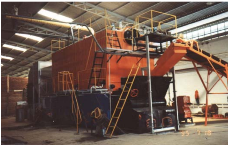
Model D-10 10ton chain grate (Indonesia)
