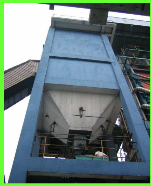
Auto ash discharge to truck
